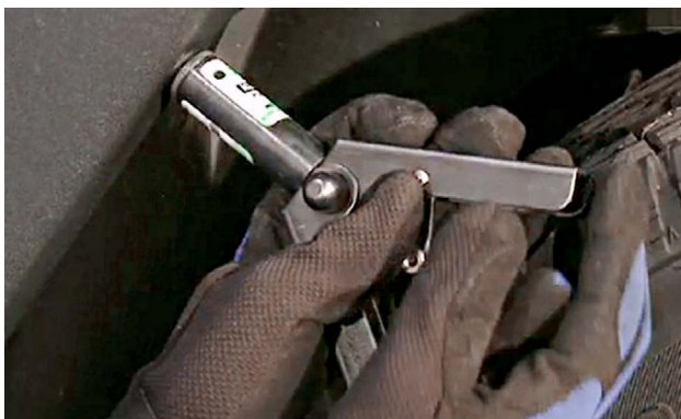
A plastic rivet tool is being used to install a new plastic rivet.
