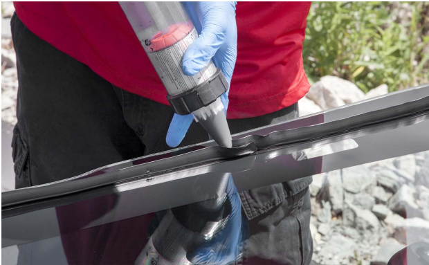
This technician is applying the urethane to the glass.
