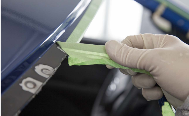
The tape that covered the new pinchweld bonding area is being pulled off after applying basecoat / clearcoat.
