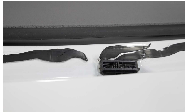
The break in the urethane bead on this pinchweld shows where adhesive failure occurred.
