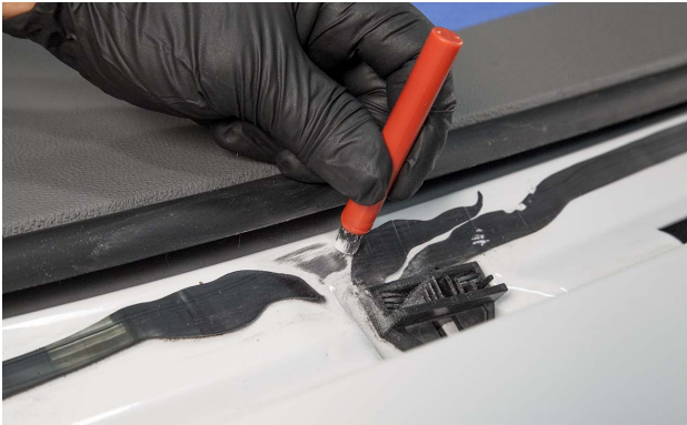
The technician is applying a one-shot pinchweld primer to bare metal on the vehicle bonding area.
