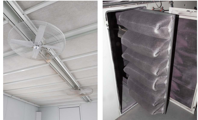
All spraybooth filters should be checked for replacement on a regular basis.
