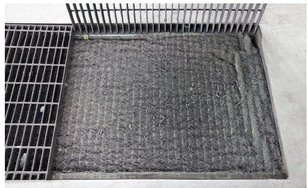
Dirty filters will restrict airflow.
