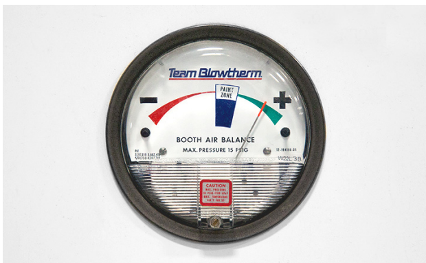
Too much incoming airflow will not evacuate dust and overspray.
