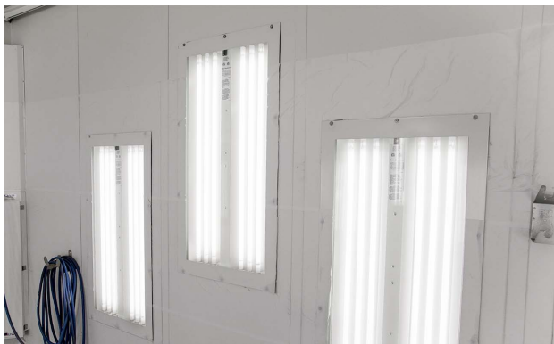
Shown are spraybooth walls that have spraybooth wrap applied.
