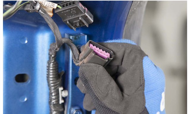
The electrical connections are being reattached on this deck lid.
