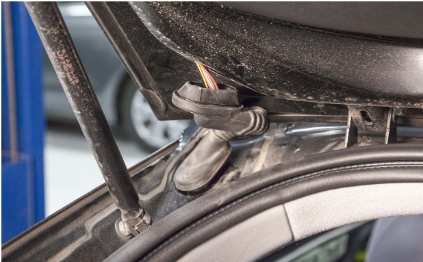
The electrical connections on a liftgate should be inspected during liftgate replacement.
