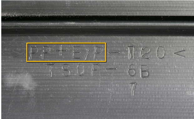
ISO codes are a standard letter code for the blend of plastic that the part is made of.
