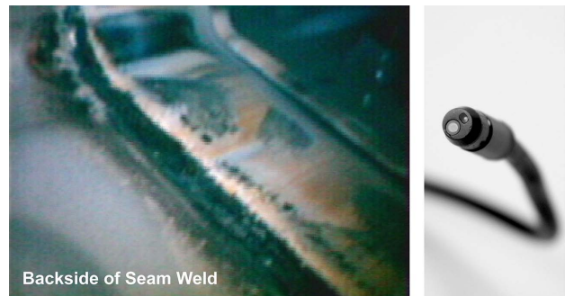
A borescope is able to display the backside of this seam weld in an enclosed area of the B-pillar.
