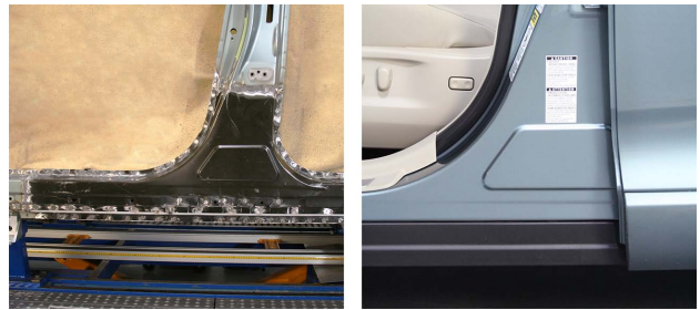
Access to the repair areas are limited after all repairs are completed
