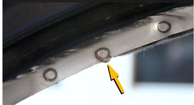
Too Close To Edge
