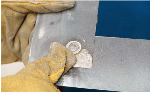
The backside of this plug weld is being inspected for evidence of penetration.
