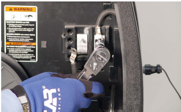
This welding machine is having the polarity switched to weld with solid electrode wire.
