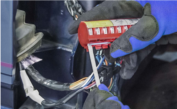
A wire loom is labeled with numbered tape for identification during installation.
