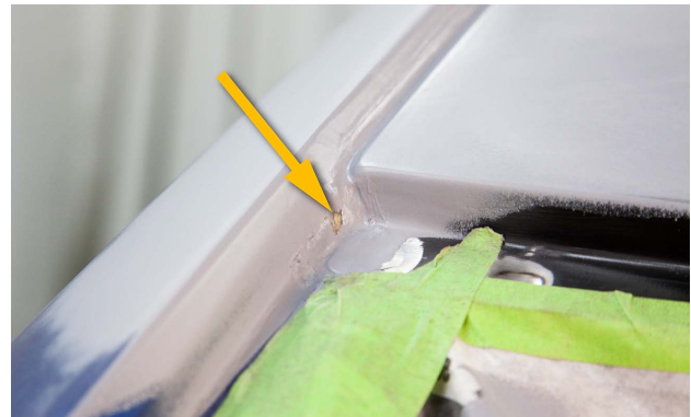
This shows a soft area of the uncured finish that easily peeled from the pinch weld.
