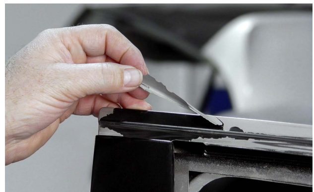
This previously refinished area has adhesion problems.
