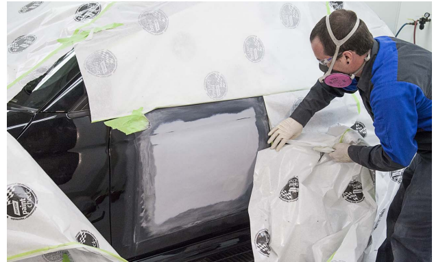
The masking tape is pulled back against itself during removal.
