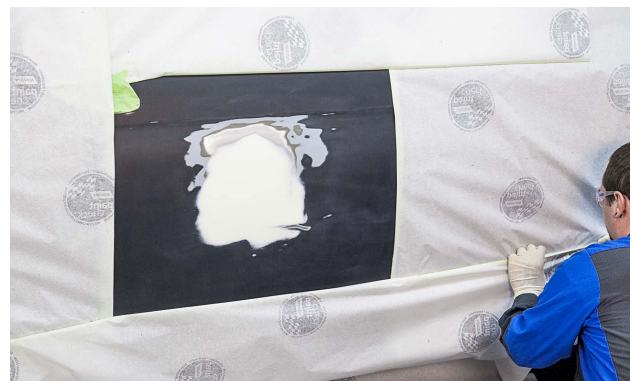
This area is being masked for primer application.
