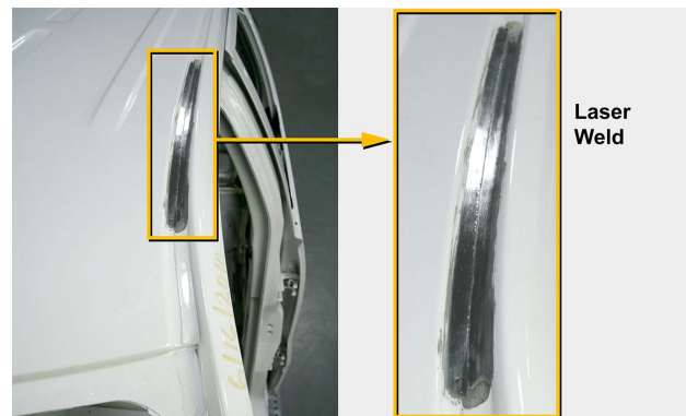
This roof panel is attached to the vehicle structure using laser welds.
