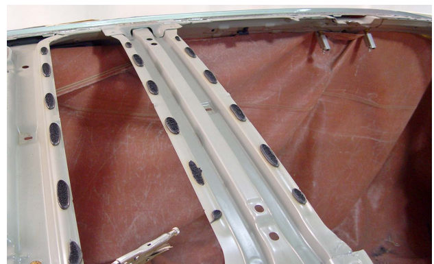
Roof bows between the B-pillars may be made of UHSS to help limit intrusion. The roof rail may be sectioned to allow adjacent panel attachment.
