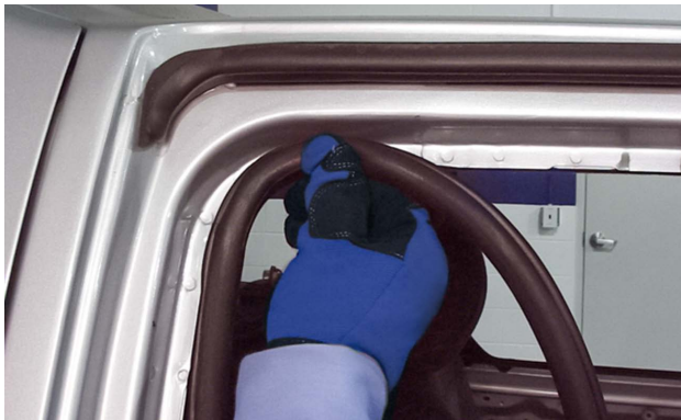
The weatherstripping is being replaced after a water leak was found.
