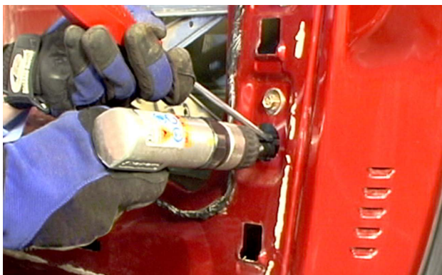
A special bit and guide tool are being used to cut the head off of the rivets used to fasten this door glass.
